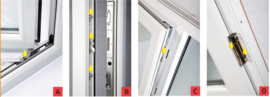
**A - Friction Adjustment Screw    C - Typical Window Lock**
